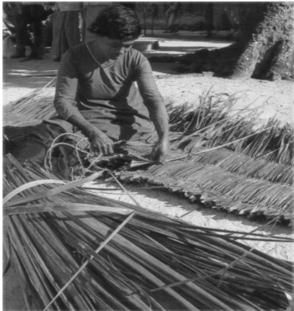
Figure 4: Weaving Palm Leaves to Create the Skin of the House
