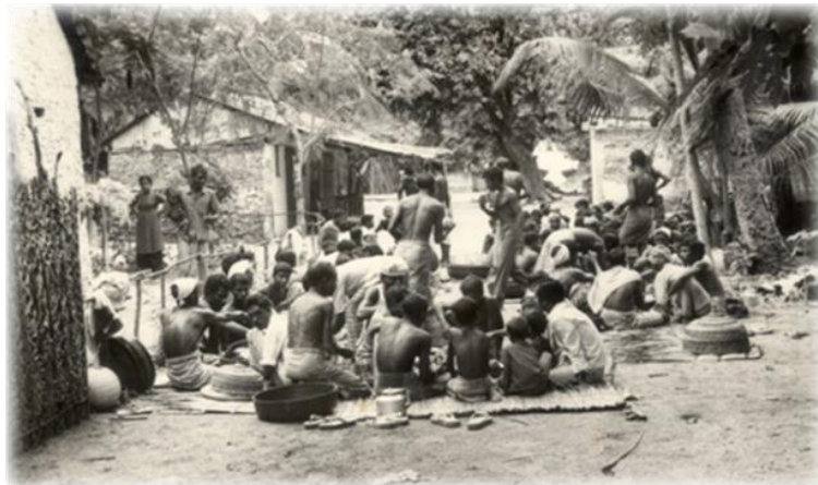
Figure 9: Working in the Outdoor Space
