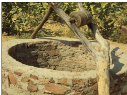
Figure 9: Kuan with a Wooden Pulley.
