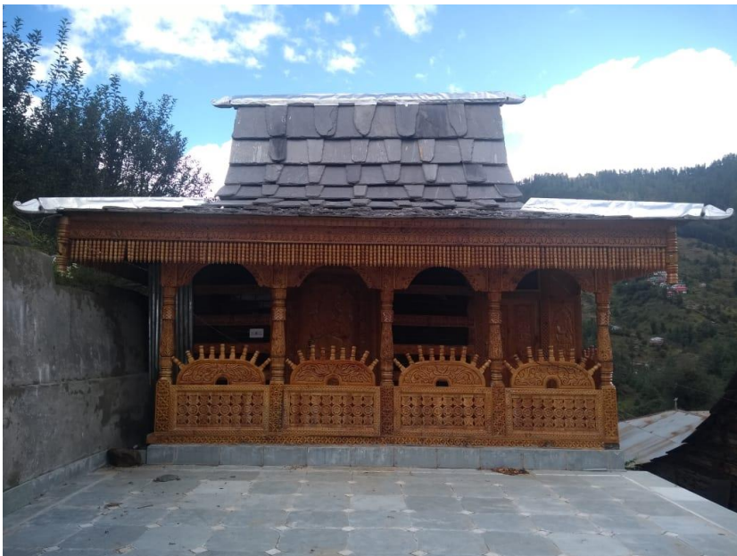
Fig. 9. Single story pent roof temple
