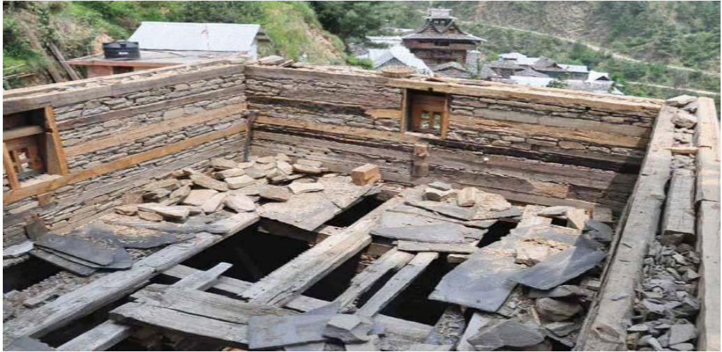
Fig. 6. Construction of Kath-Kuni walls of temple (under-construction)
